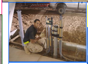
(Above and Right) The Balad team continues to set construction records.
