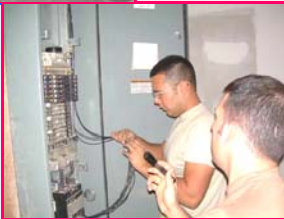
(Above) SrA Sisneros puts the finishing touch on an electric panel.
